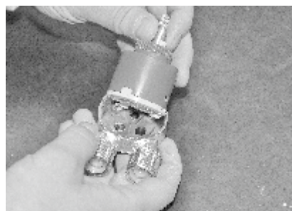
9. Pulling out the shower mixer head
