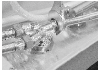
6. Detaching the water supply
