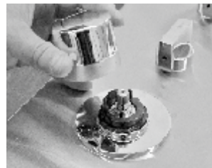
3. Removing the knob
