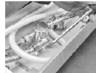
4. Detaching the water supply
