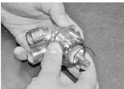
8. Unscrewing of the shower mixer head
