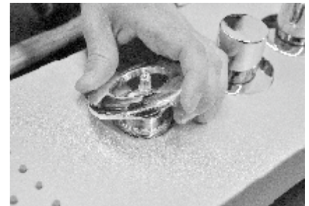
7. Removing the decorative screw on top
